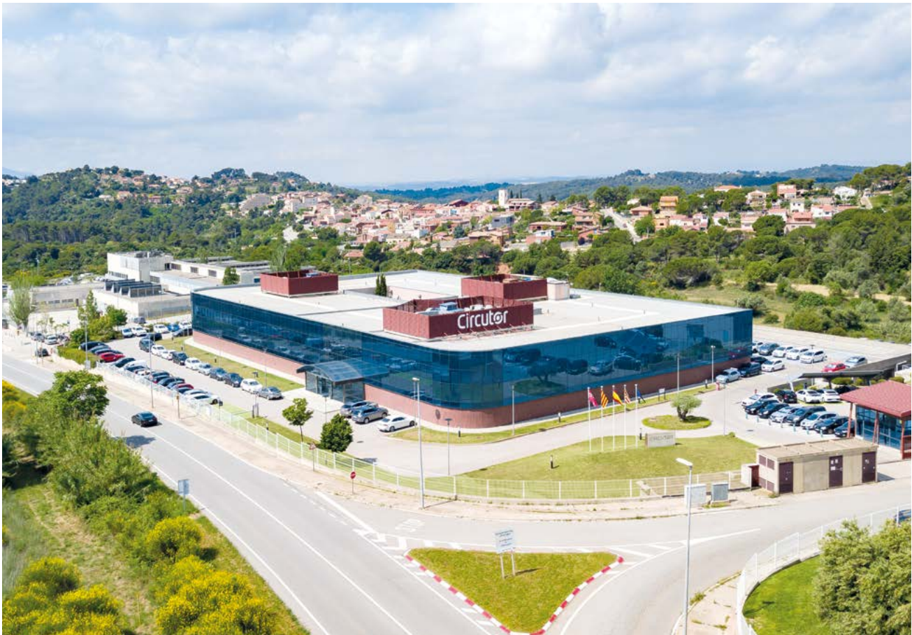
CIRCUITOR headquarters in Viladecavalls, Barcelona.
